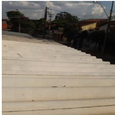
Figure 4. Roof area: natural coating, white impermeable and acrylic paintings.
